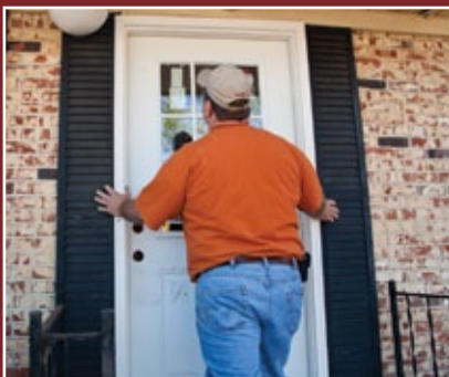
DOORS Replace faulty doors that do not seal
