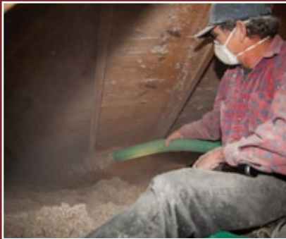
INSULATION Blow fiber insulation into the attic
